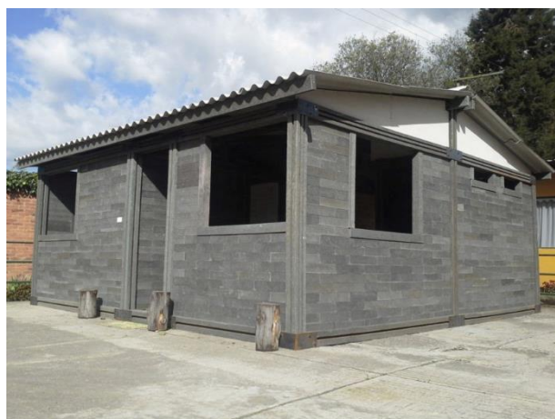
House build with recycled plastic bricks. Source: Own elaboration
